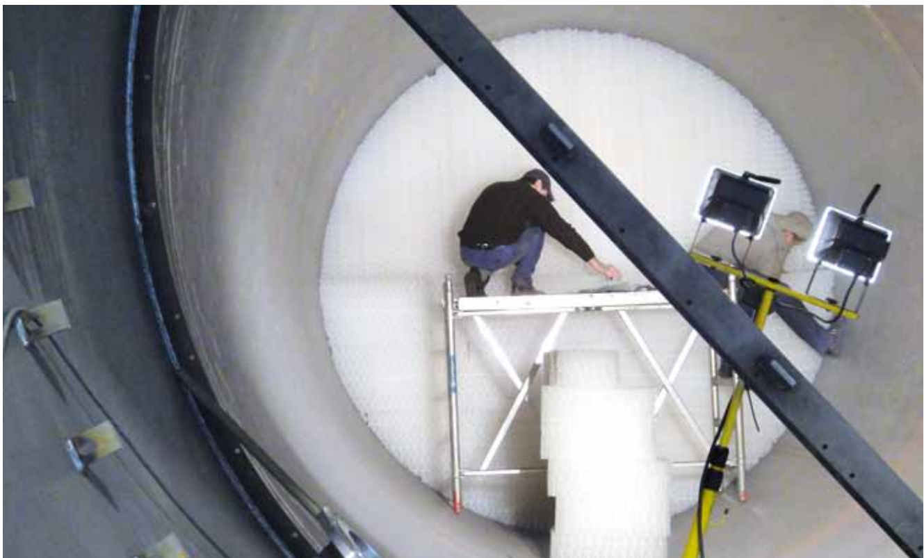
The installation of Hiflow® PLUS in a lying column at the column manufacturer's site considerably reduces transportation and installation costs at jobsite
